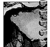
Freeze-thaw wetting/drying cracks
